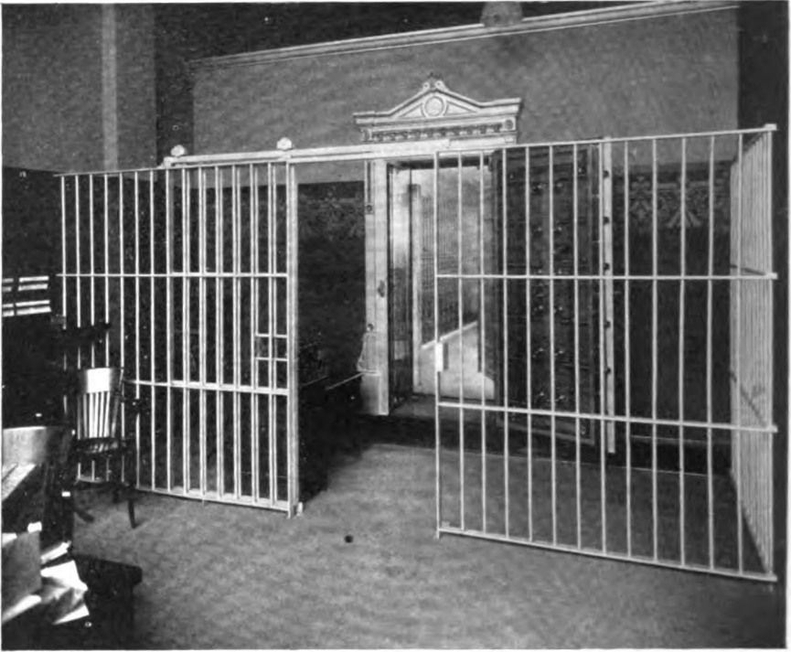
Entrance to Seattle's Only Day and Night Safe Deposit Vault
